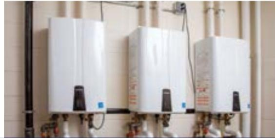
Brooks School replaced an inefficient boiler and tank system with three cascaded Navien NPE-240 water heaters.
