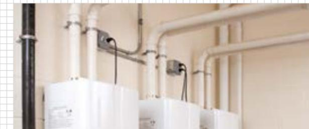
PVC venting on the Navien system is easier to install and won't corrode like metal venting.
