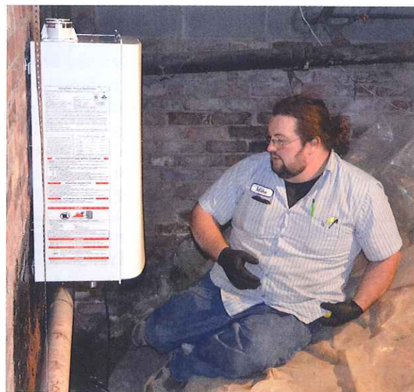
Technician from Sloan Plumbing, Greensboro, NC working on Navien tankless installation
