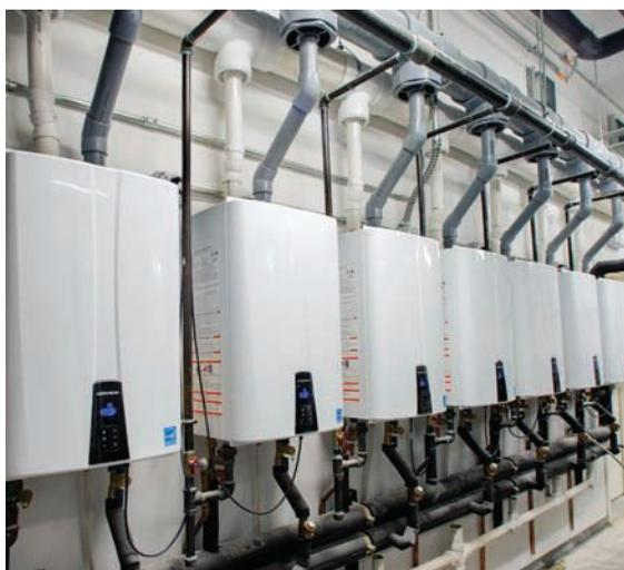
type of application. Most of us use the hot water fixture unit (HWFU) charts for specific applications and refer to the Hunters Curve for the peak gpm required for the given HWFU counts. Once we know that we can refer to the tankless unit performance specifications and determine with the required temperature rise how many tankless units will be required.
