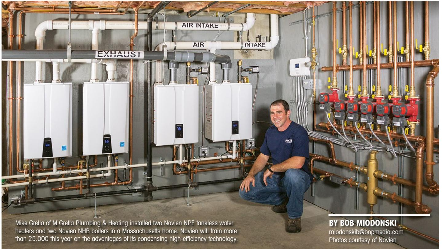
Mike Grella of M Grella Plumbing & Heating installed two Navien NPE tankless water heaters and two Navien NHB boilers in a Massachusetts home. Navien will train more than 25,000 this year on the advantages of its condensing high-efficiency technology.
