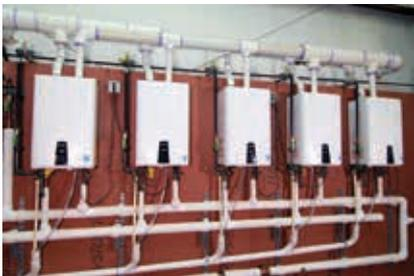
Oklahoma Textile has five cascaded Navien NPE-240As. This means the company has the ability to run a larger washer, or even a second one.
