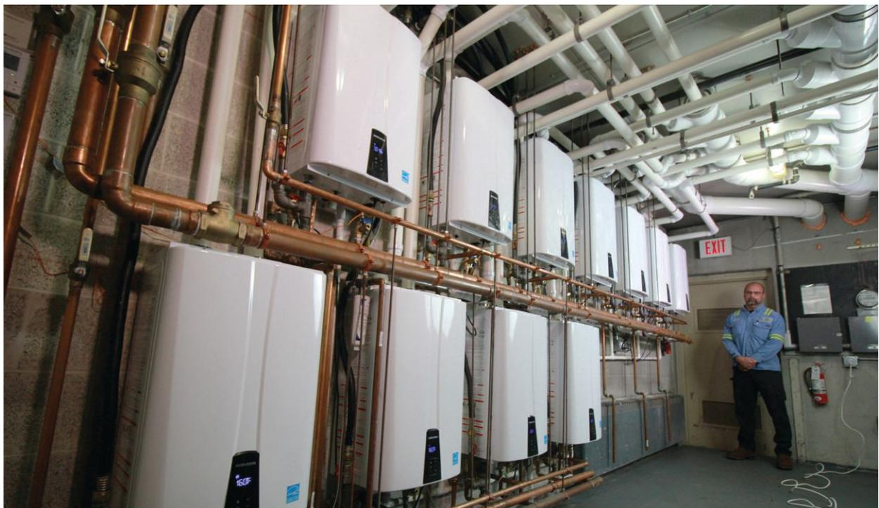
KMB Plumbing & Electrical installed 11 Navien NPE-240A units at Golden Living, a health care facility in East Stroudsburg, Penn.
