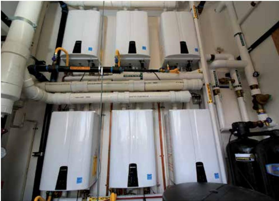
Red Robin has been proactive by installing an extra water heater at each of its facilities. At the Lakewood location, six were installed and piped in parallel allowing for redundancy.
